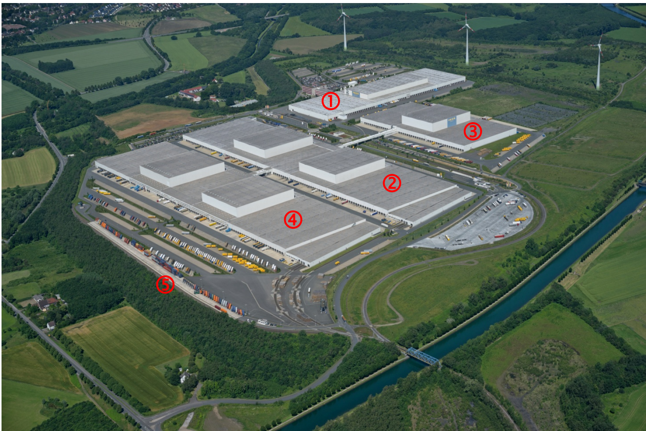
View of the IKEA distribution centre Dortmund-Ellinghausen from south-east: In the background the Customer Distribution Centre (①), in the front (②, ③ and ④) the three sections designed to supply the European stores. In the utmost southern part of the site (⑤) the container transshipment area (Picture: IKEA Distribution Services GmbH & Co. KG, June 2014)
